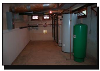
Figure 3—The hot water storage and expansion tanks are in the basement of one of the bunkhouse cabins.
