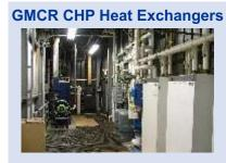
wash water for processing and other building uses. An air/water heat exchanger on the engine exhaust preheats water in the building's hydronic space heating system.
